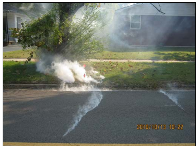
Inflow source identified during smoke testing
